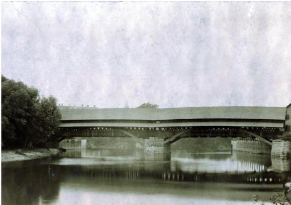
This 1894 photo shows the original South Channel Bridge just after it was reinforced to accommodate a new trolley line. This span was severely damaged by the December freshet of 1901 and was replaced by a new steel bridge in 1904.
